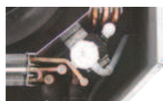
Condensate pump integrated in all sizes
